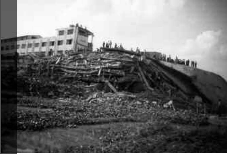
Collapsed Spectrum Garment factory in Savar, Bangladesh
